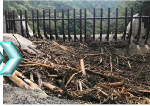
図-6 流木捕捉後
