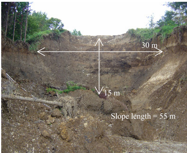
Fig. 12 A deep-seated landslide that occurred in the Senokuchi area, Taketa, Oita Prefecture, on 6 September 2005.
