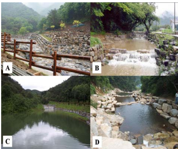
Fig. 13 Torrent erosion control (A), small sub-stream maintenance (B), water reservoir (C), and step-type water storage dam (D) using natural materials.
