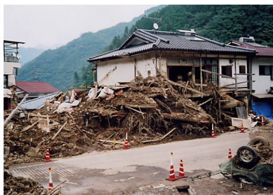
Photo 11 A debris flow at Kamishiiba, Shiiba Village.
