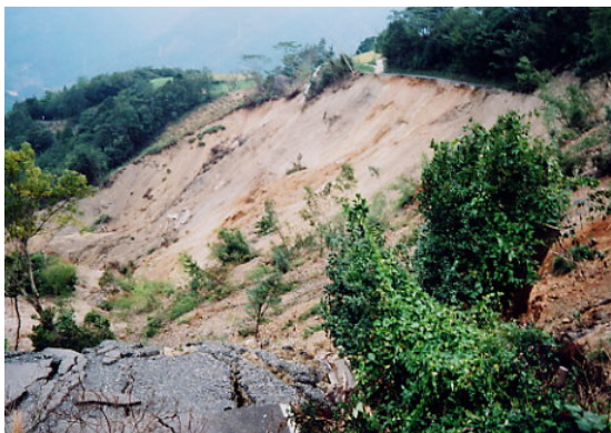
Photo 1 A large slope-collapse at Koba in Shiiba Village.
