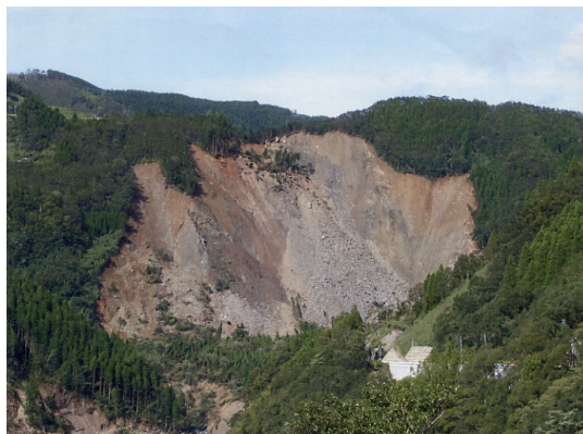
Photo 5 A large slope-collapse at Nonoo in Saigo Village.
