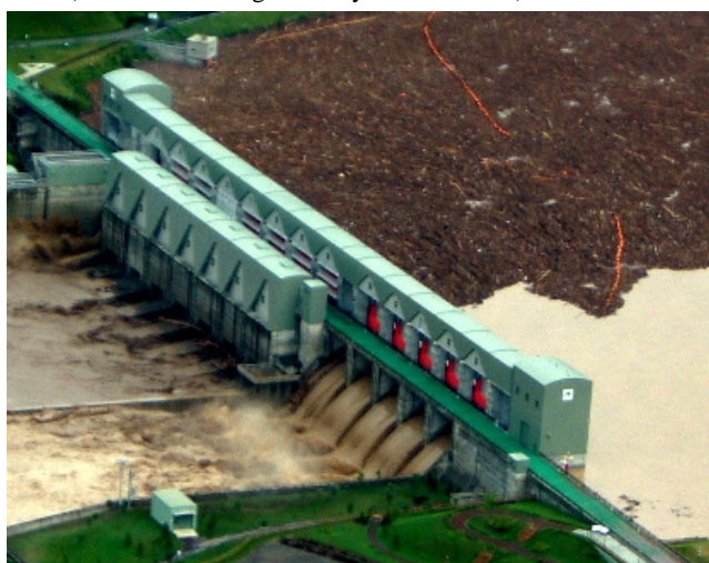
Photo.2 50,000 m 3 of drift wood accumulated in the Nibutani dam reservoir (taken on 10 th Aug. 2003 by the Hokkaido development bureau)
