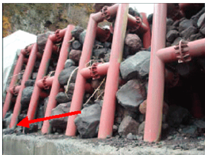
Photo 3 Steel pipe SABO dam (open type) trapped large rocks of debris flow at Rishiri island in 2007.
