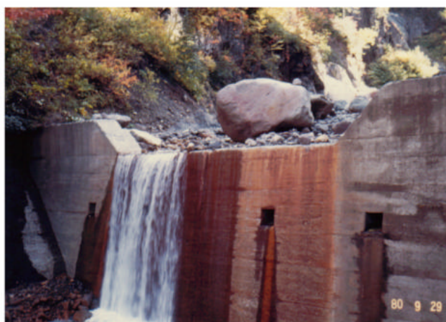
Photo 2 Concrete SABO dam (closed type)
