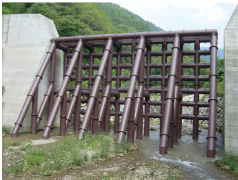
Photo 4 Steel pipe SABO dam as downstream end structure of debris flow torrent. Its opening is small, almost equal to a diameter of the rocks transported at the front part of debris flow.
