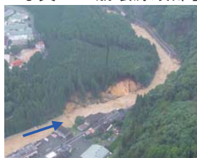
写真-2 河岸侵食崩壊 [星野川本川]
