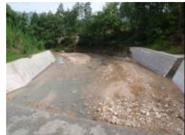
(c)最下流部の床固工の状況
