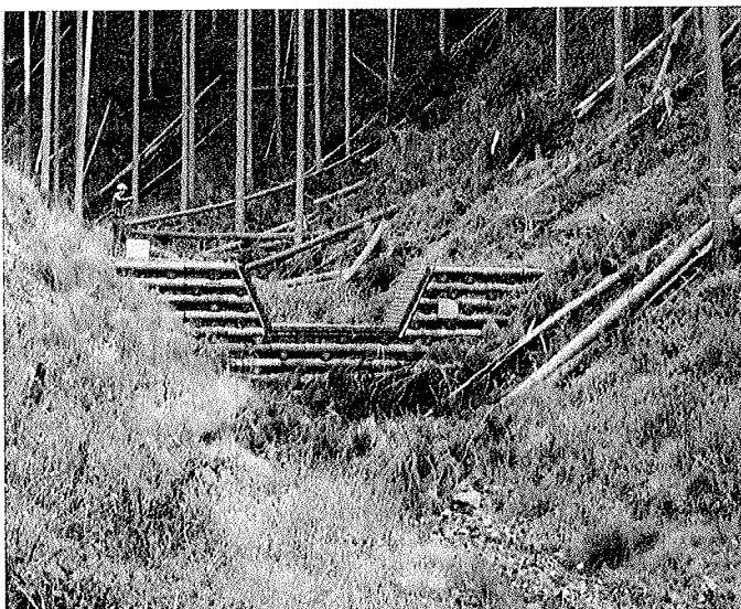
Photo.1 Wooden dam built in field
